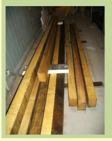
The new timber that will provide additional strength and support in the roof have arrived and work has started in preparing these for installation.
